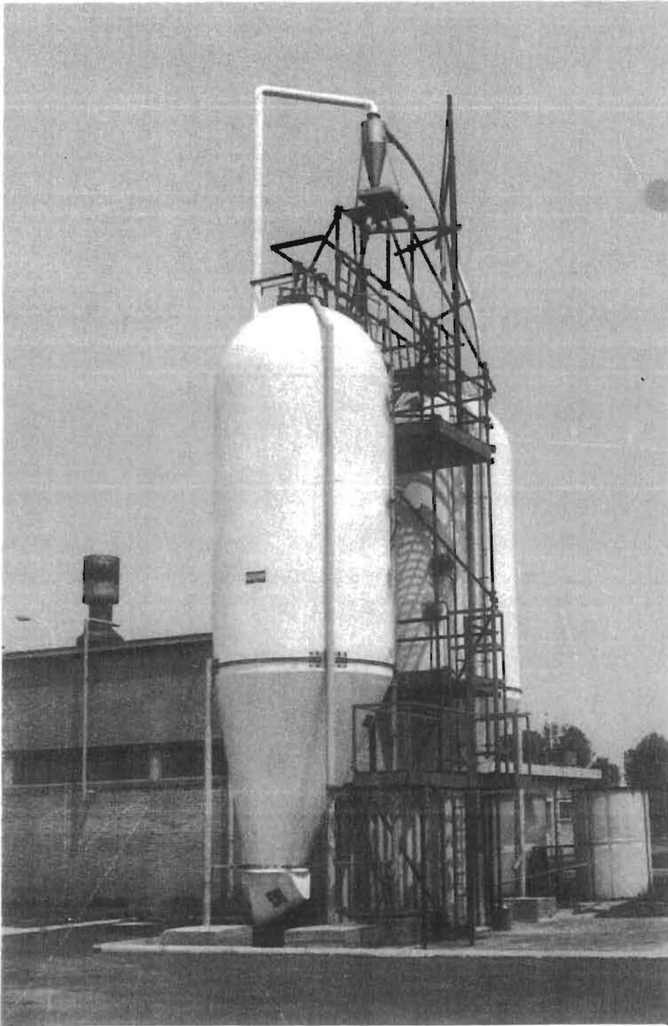
Fig.5. Fiber-glass midi-silos for controlled atmosphere storage trials at pilot scale.
