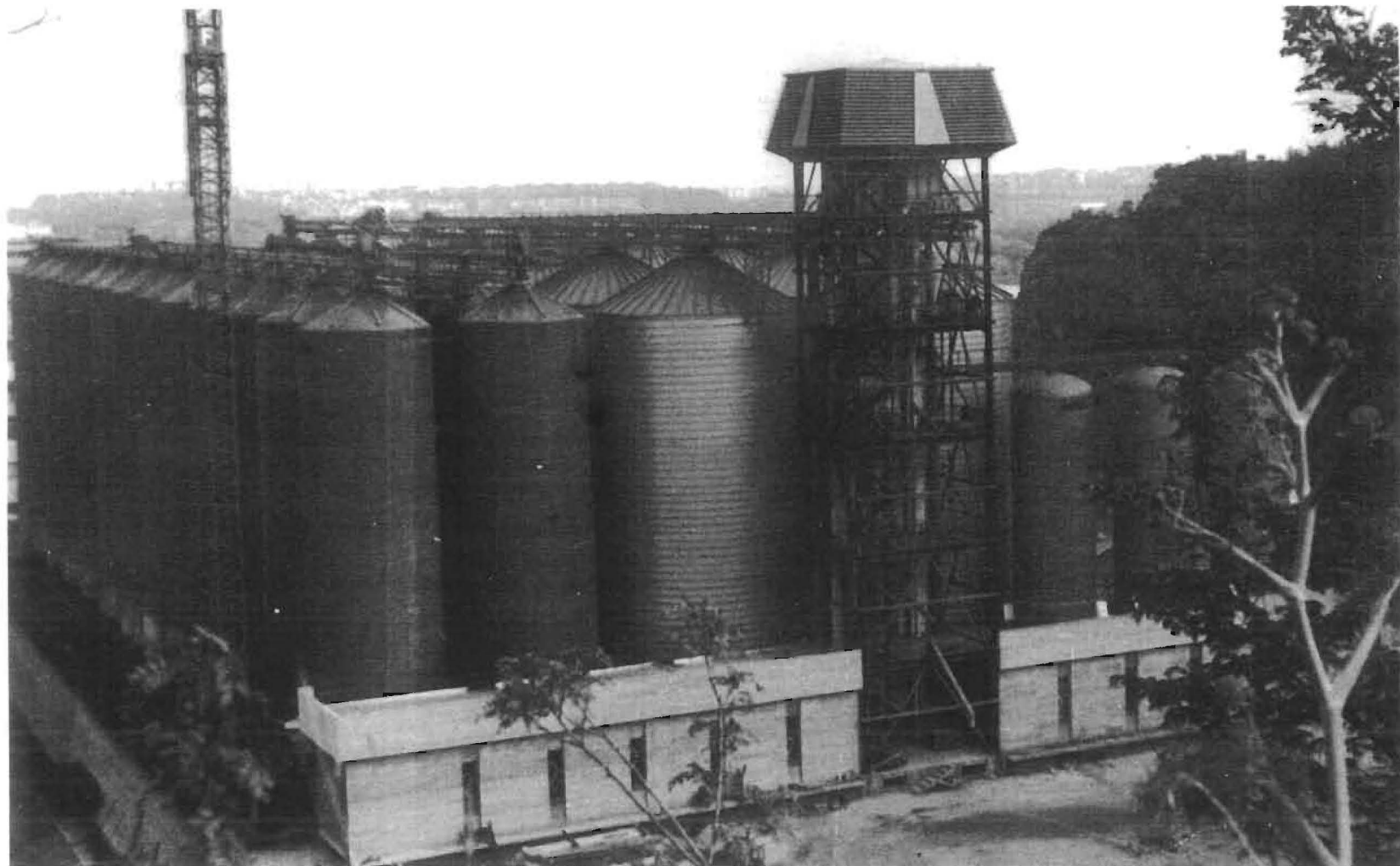
Fig.8. Silo 3 of Società Romana di Macinazione, Rome, for the storage of wheat. The fiber-glass bins (600 m 3 each) are equipped for nitrogen fumigation and storage of grain.
