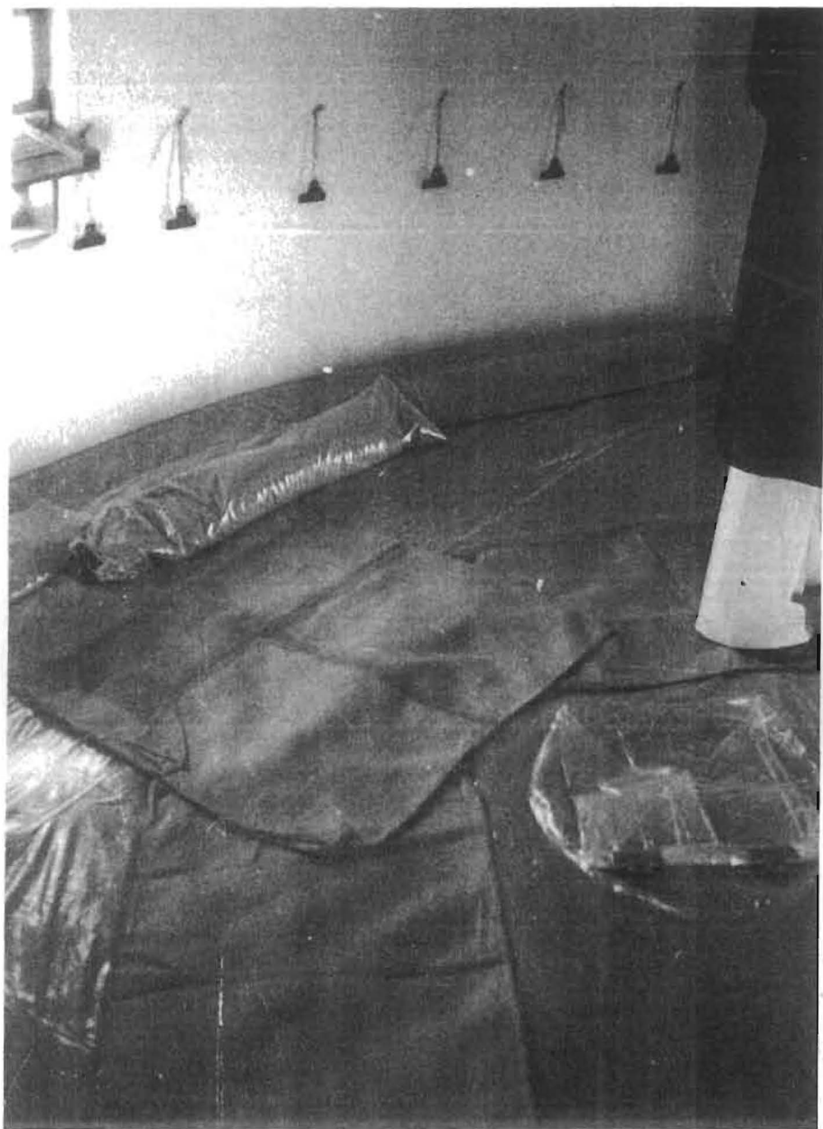
Fig. 3. Interior of clay/straw walled silo with the grain covered with polyethylene (to prevent air exchange and prevent the grain from warming up).
