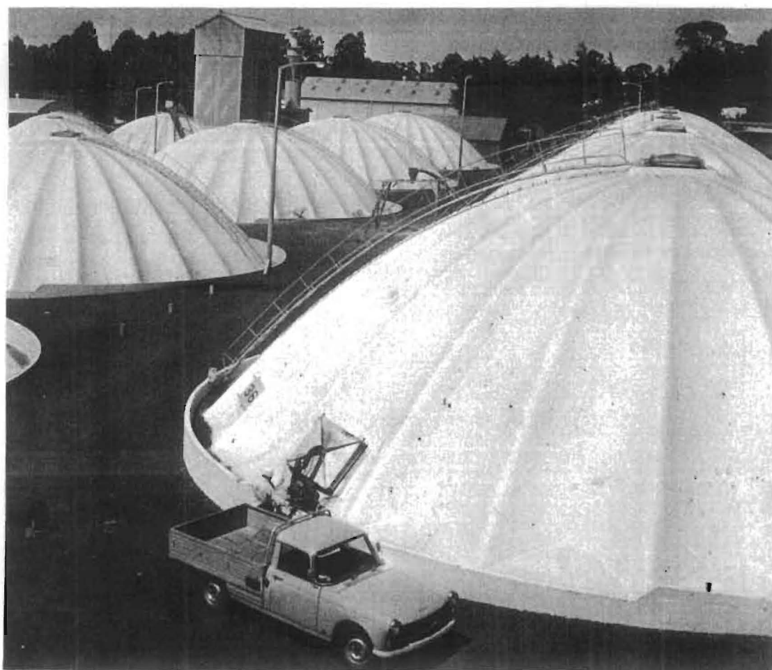
Fig. 1. View of the "Cyprus" bins at Kitale. In the foreground, a bin is being pressure tested for leaks.
