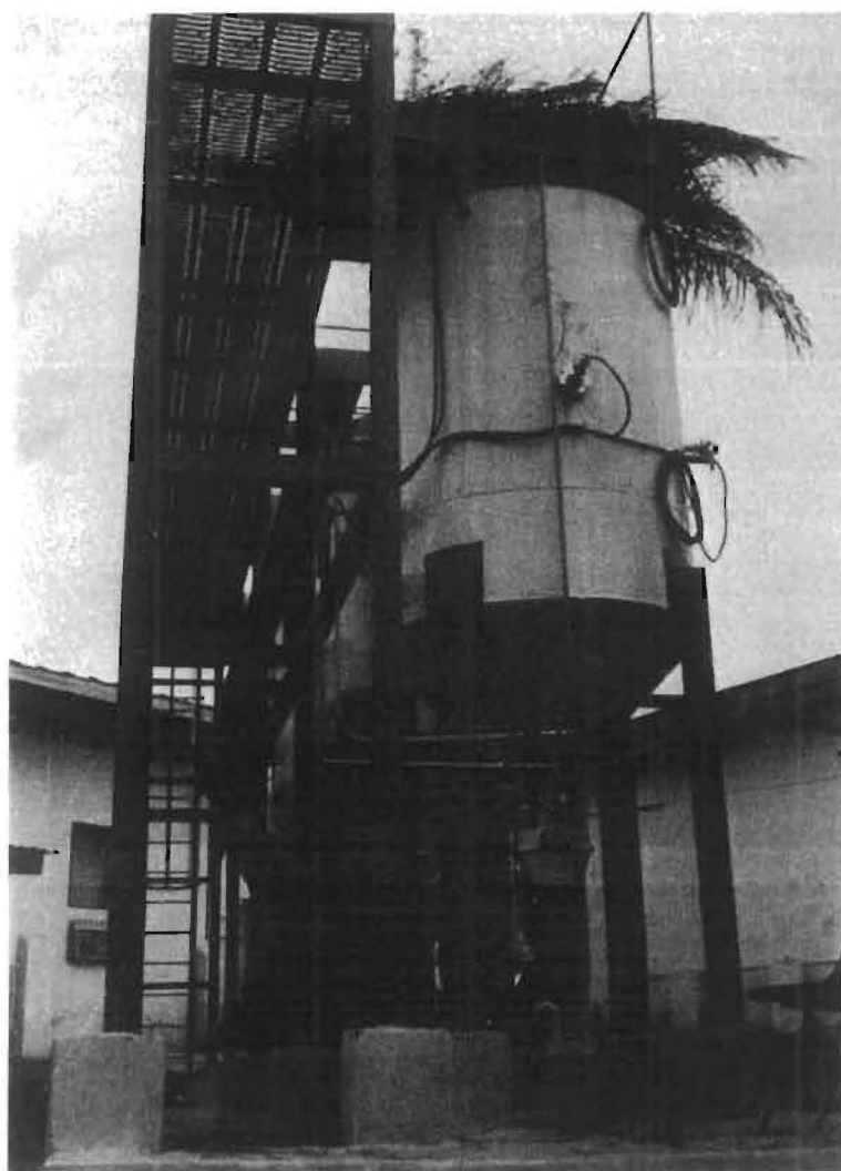
Fig.7. Experimental shaded steel bin at NSPRI, Ibadan. Simple shading of the roof of an airtight metal bin, leaving enough space between the thatch of palm leaves and the top of the storage structure to ensure free air circulation, permits safe storage of grain in a nitrogen atmosphere.
