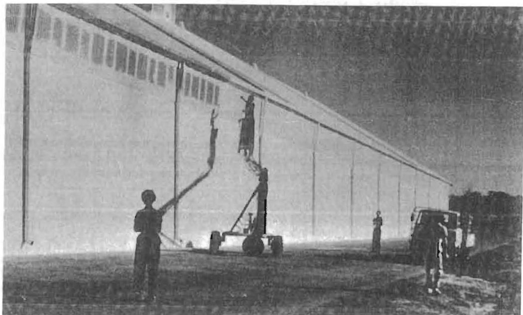
Photo 6. Application of final coat of reflectant material over previously sealed roof and wall at Meckering.
