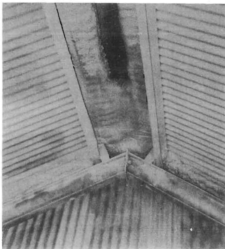
Photo 11. Sealing inside the roof ridge line of a horizontal storage.
