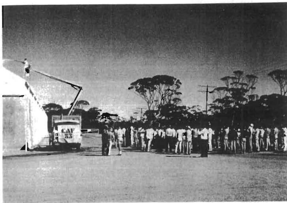
Figure 1. Detergent solution being applied to the roof of a newly sealed storage.
