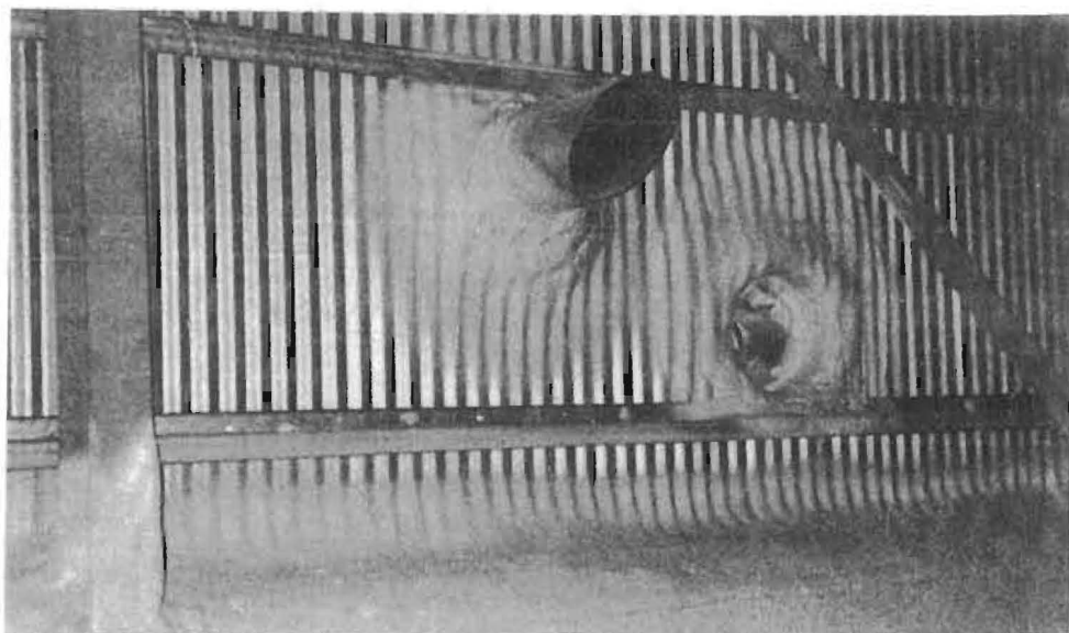
Photo 10. Foam application along an inside wall ledge and around the fan and pressure release duct fitted into a gable and wall.
