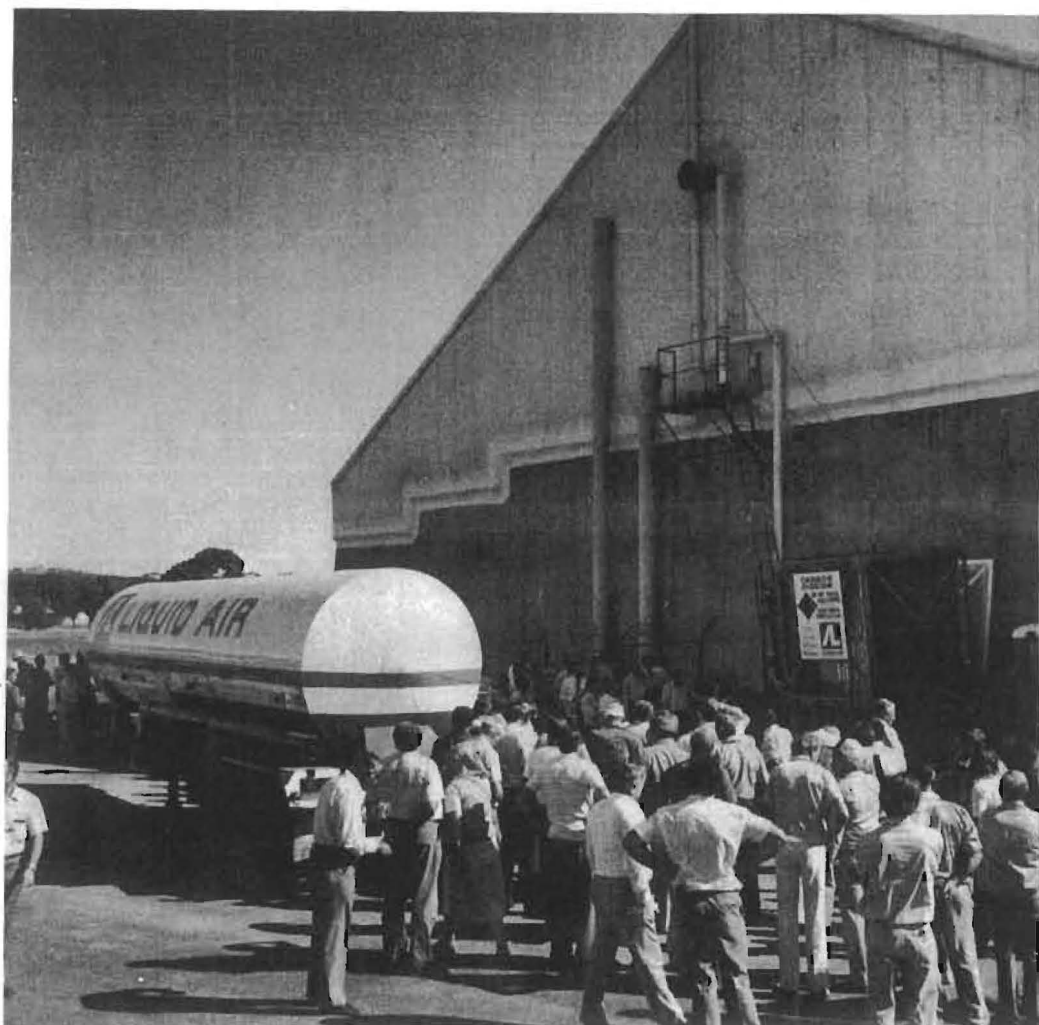
Photo 23. Demonstration of the introduction of \text{CO}_2 gas into a sealed storage at Cunderedin. Liquified carbon dioxide is supplied by tanker from where it is pumped through a vaporiser into the storage.
