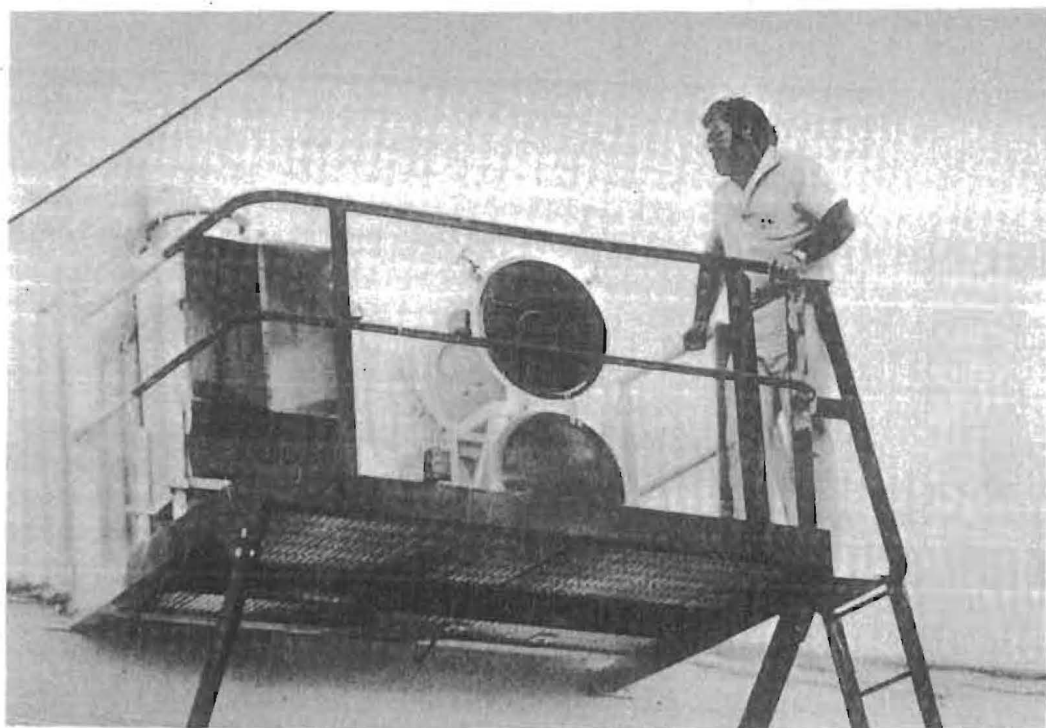
Photo 12. Pressure relief vent and fan built into gable end wall of horizontal storage at Kellerberrin. The fan cover is opened while pressurising the storage and is sealed for the pressure decay and leak detection test.
