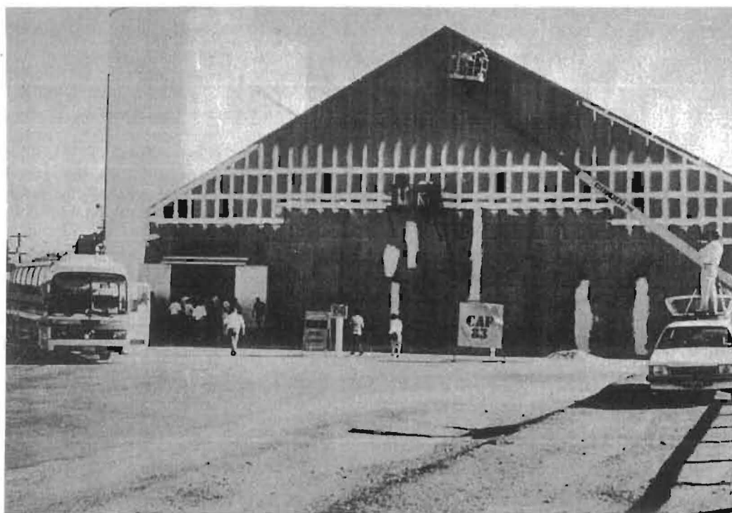
Photo 4. Sealing in progress on the end wall of a horizontal silo at Meckering. Note all lap ends of the corrugated iron sheets used to clad the gable-end wall are individually sealed, as are surface cracks evident in the concrete wall.
