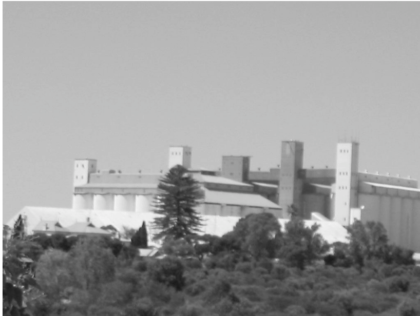
Figure 1. The 2000-tonne sealed concrete vertical silos at AusBulk Wallaroo grain terminal.
