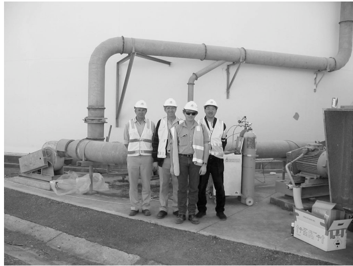
Figure 6. Close view of the HDS-80 setup.
