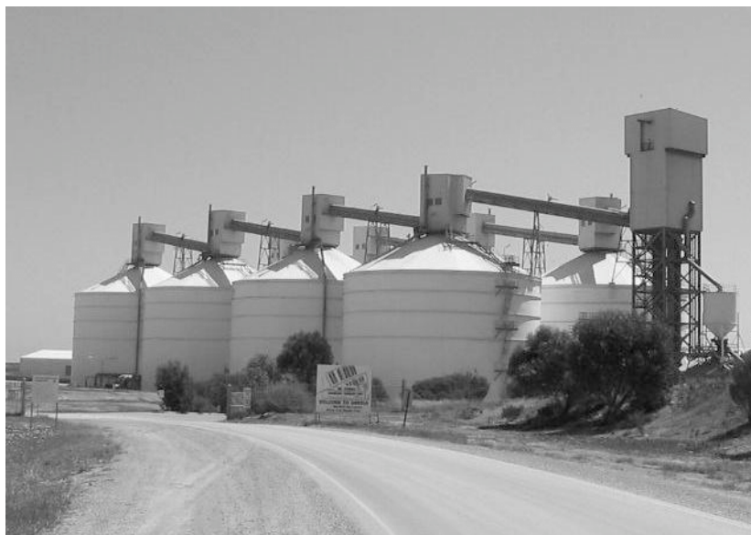
Figure 2. The 10000-tonne welded steel squat silos at AusBulk Wallaroo grain terminal.
