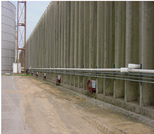
Figure 2. Left photo shows closed loop fumigation (CLF) system PVC pressure piping system above aeration fans along one side. Right --CLF fan, suction pipe from roof and pressure pipe.
