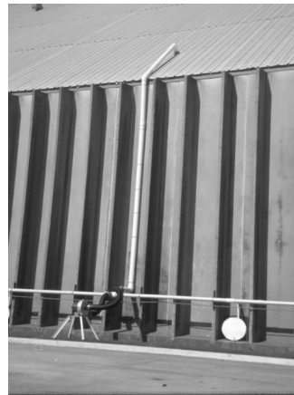
Figure 2. Left photo shows closed loop fumigation (CLF) system PVC pressure piping system above aeration fans along one side. Right --CLF fan, suction pipe from roof and pressure pipe.
