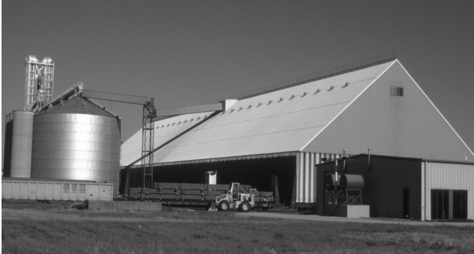
Figure 1. Peavey Company's 3.3 million bushel warehouse at Tulsa Port of Catoosa, showing concrete silos and steel bins. Company installed CLF system in warehouse in 2000.
