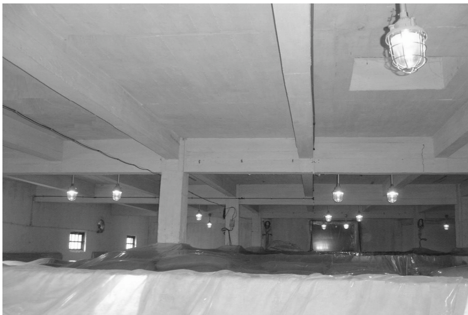
Picture 1. Inside view of the bag-stacked warehouse
