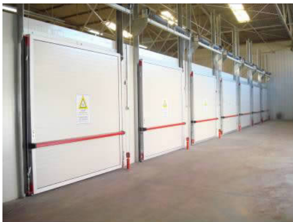
Fig. 3 CA facility in Greece (total 1029 m 3 treatment rooms)
