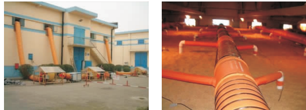
Fig 1 Photographs of portable ventilation system for in – store drying
