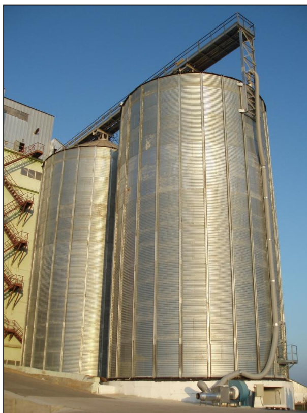
Fig. 1- Metal bin equipped with phosphine recirculation system.
