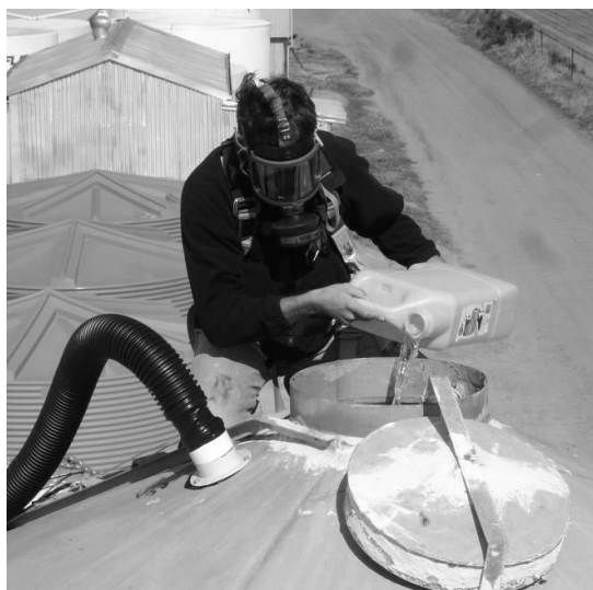
Fig. 2- Pouring liquid Ethyl Formate into the top of the silo.
