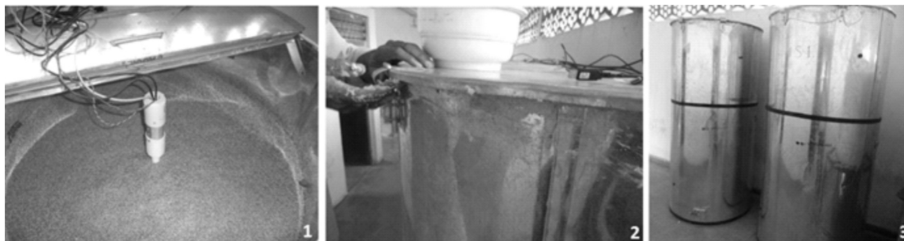
Fig. 5. Sensor rod installation 1 , sealing of leak points - joints with wheat flour paste 2 and final experimental setup 3 of the steel bins.
